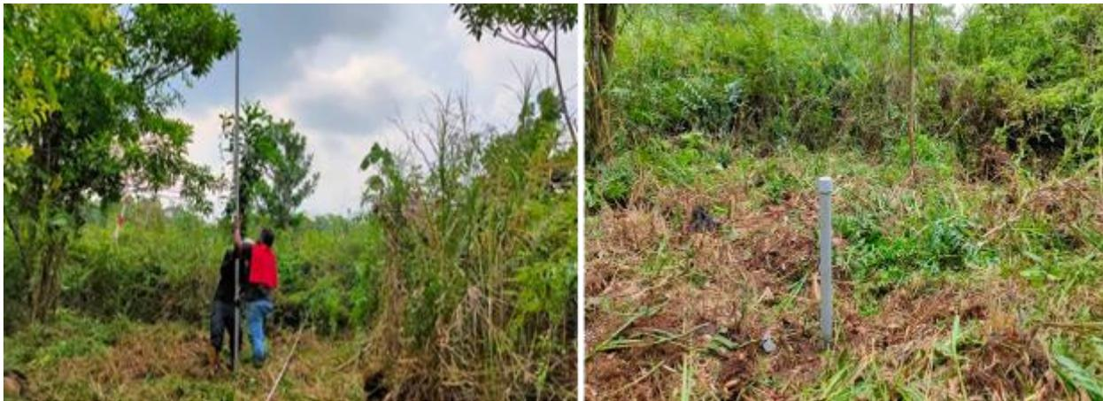
**Figure 9.** The installation of 4 units of piezometers at FC 25 and 38 of Bukit Belata (Ext.) Forest Reserve
